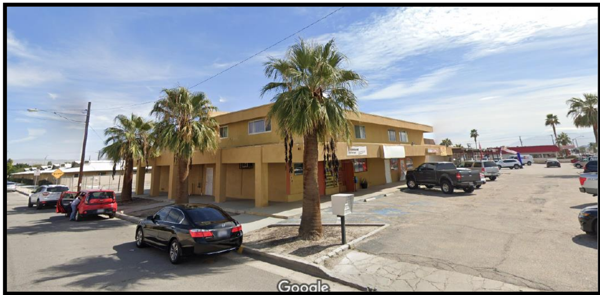
Cairo Avenue Frontage
